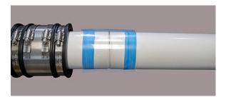
4. Center the FEP liner over the pipe ends and PTFE tape.
