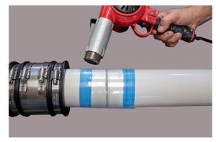
5. Use a heat gun to shrink the FEP liner to the pipe.
