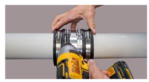
6. Center the coupling and tighten the bands.
